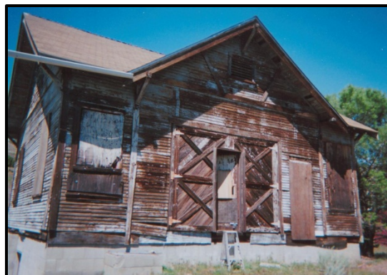
Leona Valley Schoolhouse, Leona Valley, Los Angeles County.
