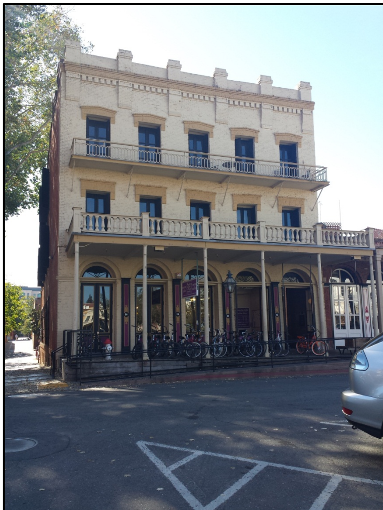
Vernon-Brannan House, Sacramento, Sacramento County.
