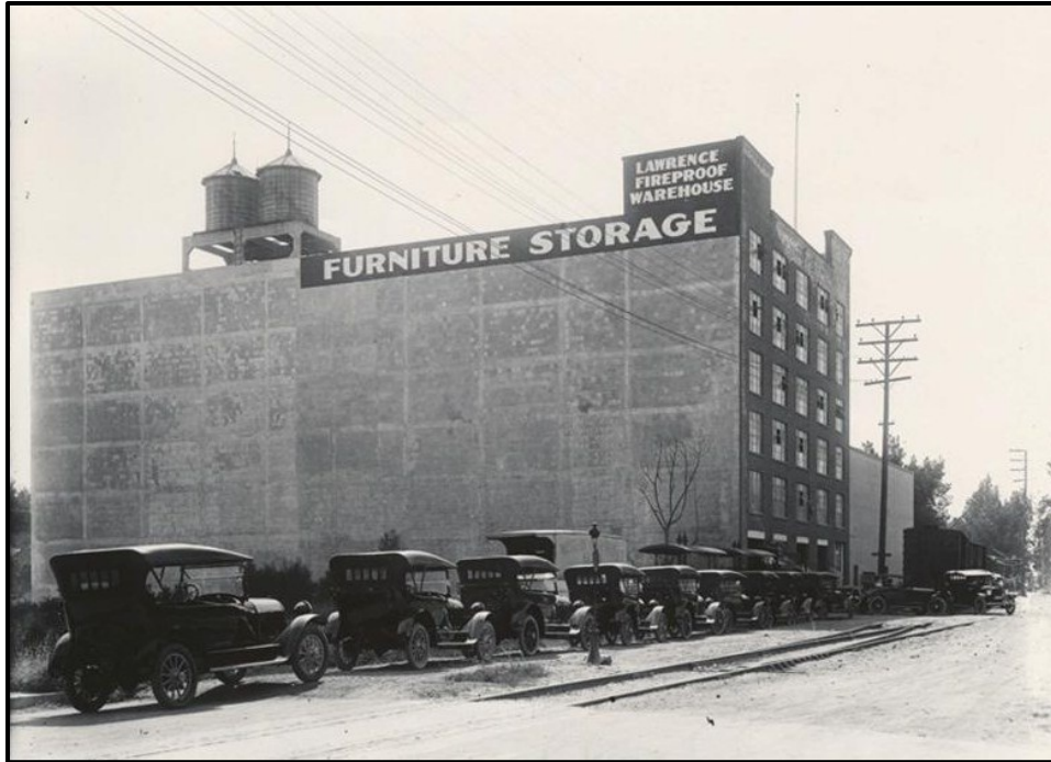
Lawrence Warehouse, Sacramento, Sacramento County.
